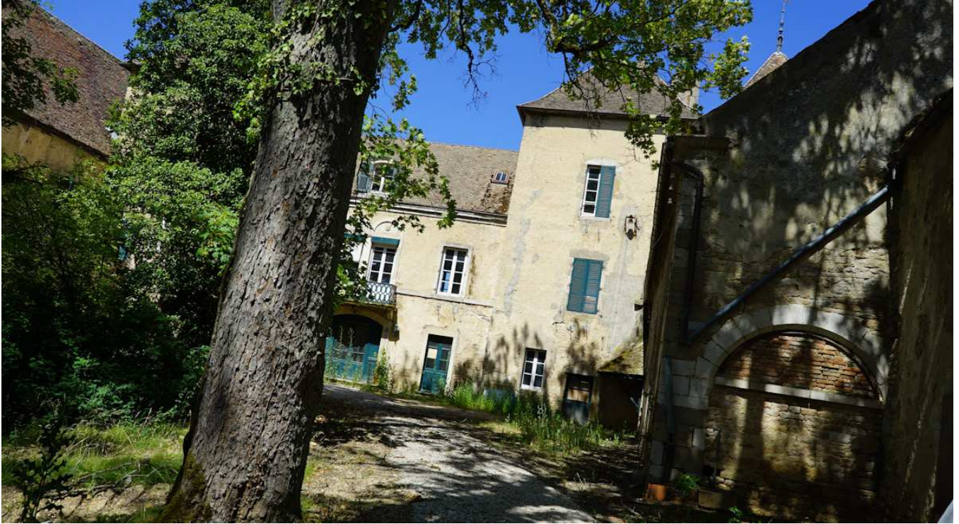
The main building seen from the village side
